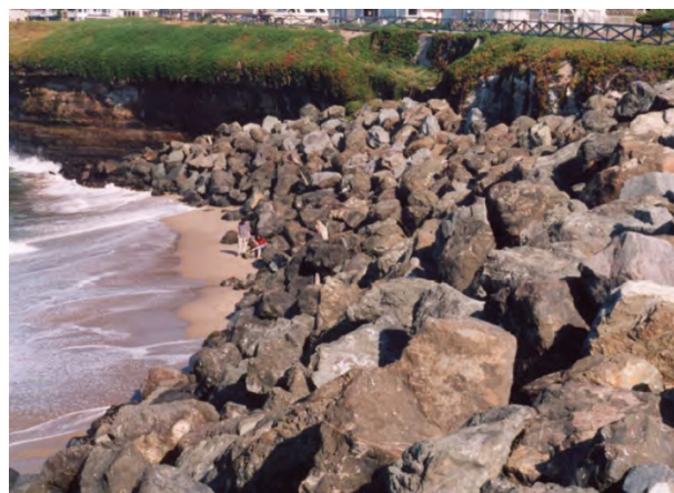
FIGURE 1. Revetment in the city of Santa Cruz showing placement loss eliminating nearly the entire beach. 26
