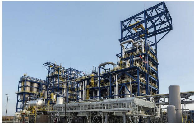
Monolith's current Olive Creek production site
